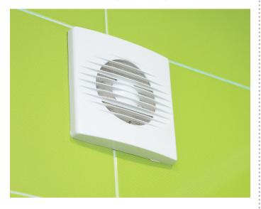
ventilation systems pull fresh air into the property through background vents and expel moist and polluted internal air out of the property through extract fans.
