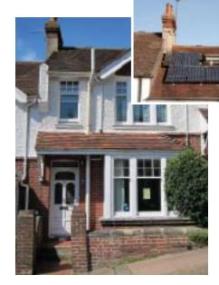
This building demonstrates how far emissions can be reduced for a simple house, by employing the most cost-effective measures. Solar panels for hot water were installed several years ago, along with a highly insulated hot water tank.
