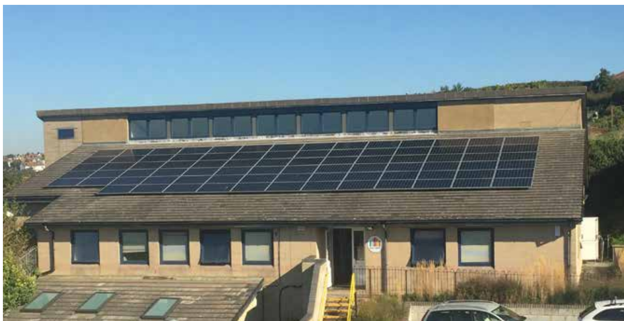
St John's College Brighton, showing the completed PV system installed in 2018
