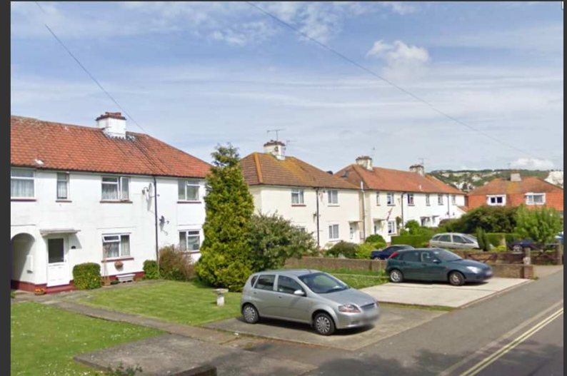
Biomass boiler plant
