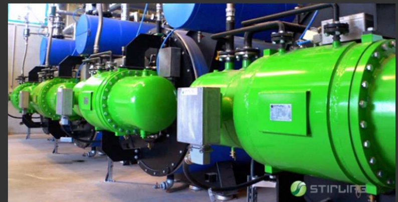
Gasified Woodchip fired CHP
